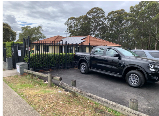
Figure 4: View of administration building, facing south-east from neighbouring carpark.
