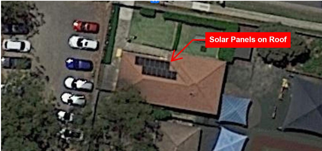
Figure 6-1: PV Cells on Roof (google maps satellite view)
